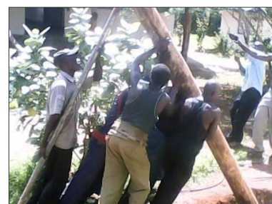
Installation of electricity power by the power company
